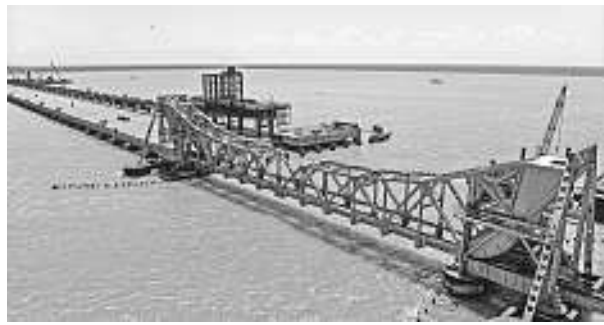
A view of the new Pamban bridge on Saturday. PTI
